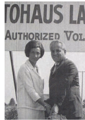
Herbert W. Wanner and Marianne Wanner at the groundbreaking of the Route 72 showroom, 1966
